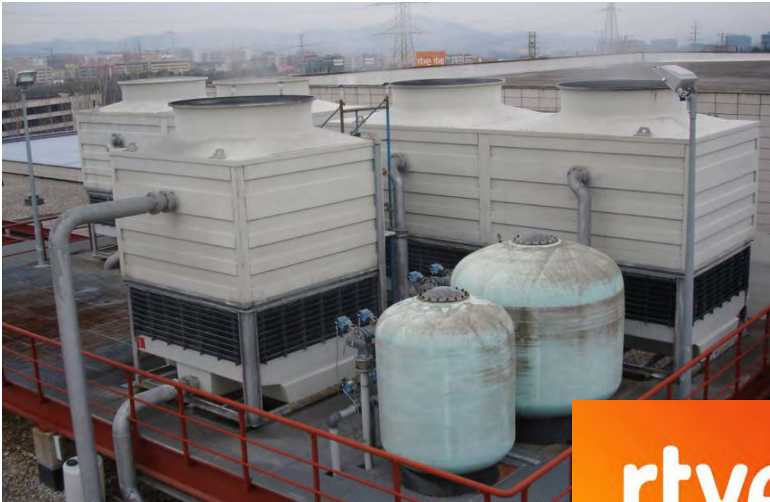
SPANISH TELEVISION RADIO Sant Cugat del Vallés (Barcelona) 3 Cooling towers Total: 5 MW
