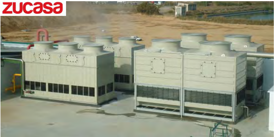
ZUMOS CATALANOARAGONESES, S.A. Fraga (Huesca) 2 cooling towers 2 NH3 evaporative condensers Total: 5 MW
