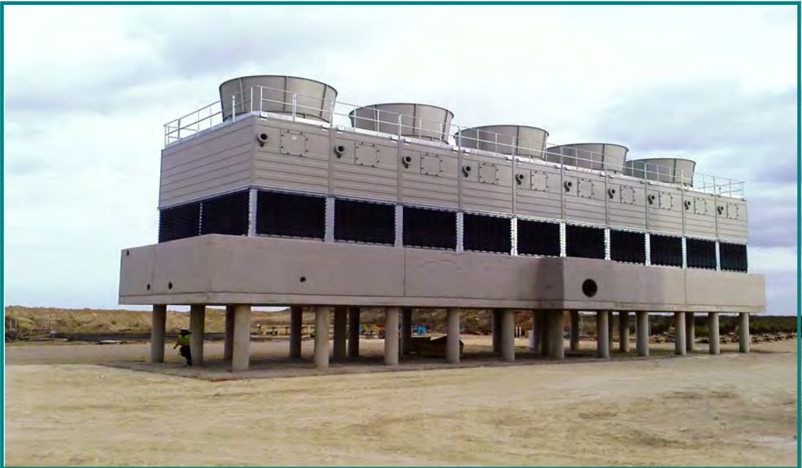
Biomass Plant Briviescas (Burgos) 5 cells of 5,000 kW each Total 25 MW
