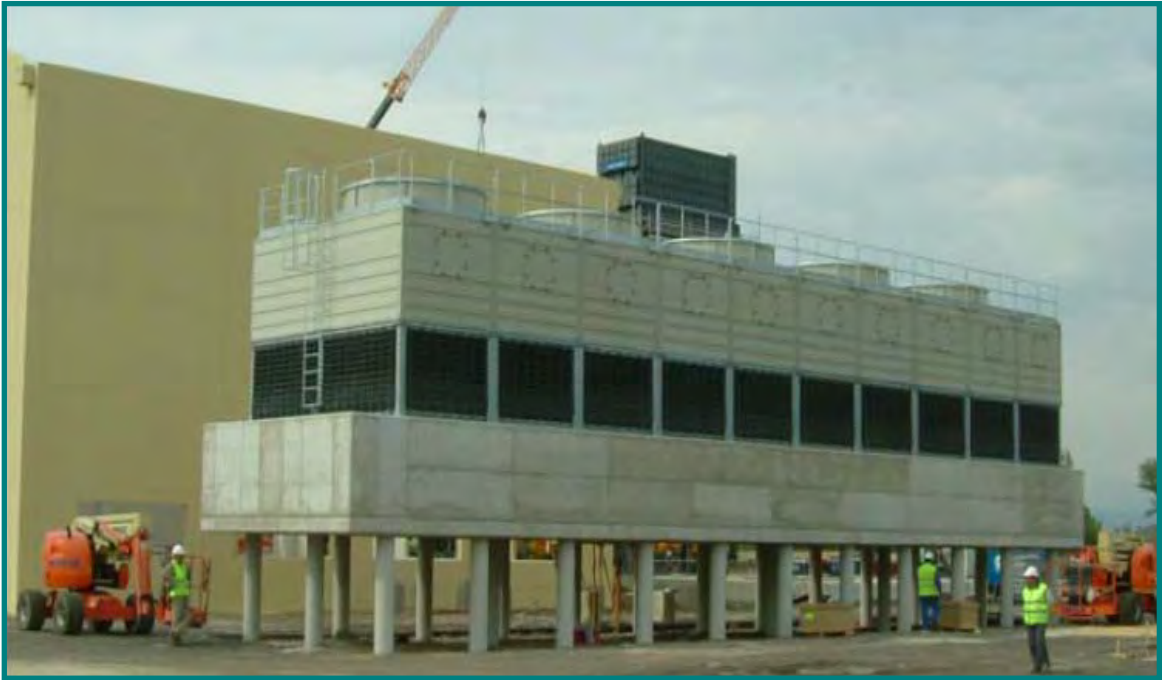
Biomass Plant Briviescas (Burgos) 5 cells of 5,000 kW each Total 25 MW
