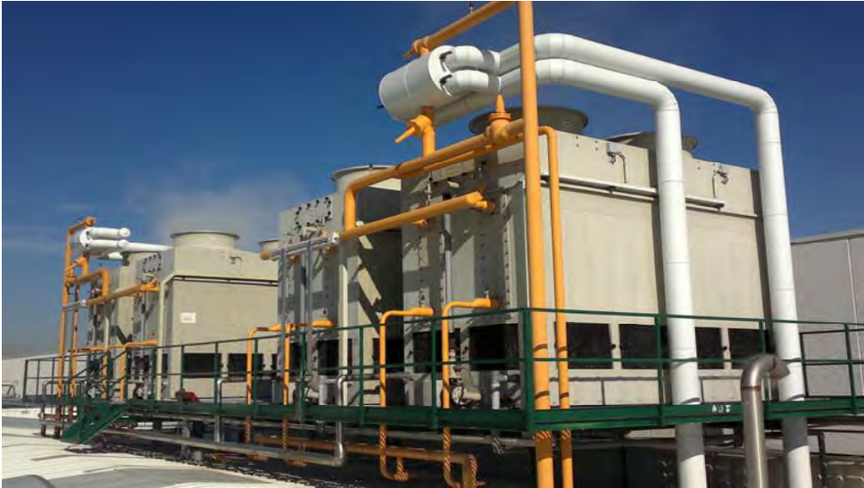
CHEESE ENTREPINARES Santovenia de Pisuerga (Valladolid) 4 NH3 evaporative condensers Total: 3.2 MW
