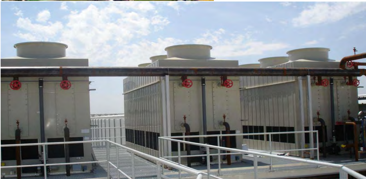
Guissona (Lleida) 4 NH 3 evaporative condensers Total: 4.0 MW
